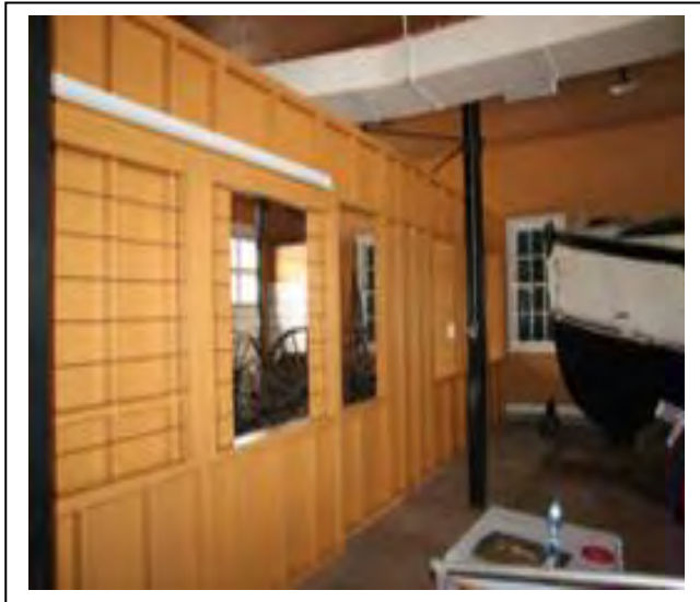
Beginning of the construction of the wire system.
